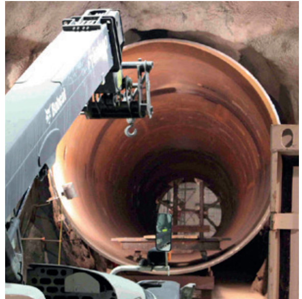
On-site installation of the fabricated components
