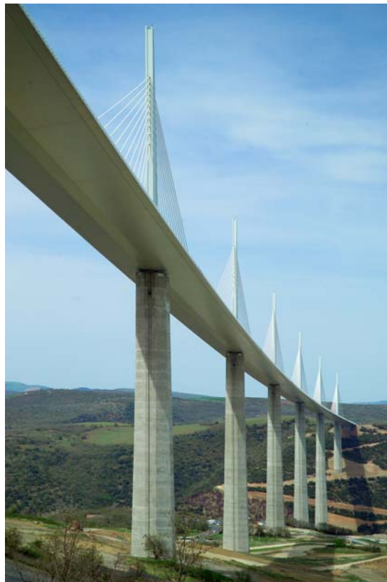
Figure 21 : The Millau Viaduct after completion
