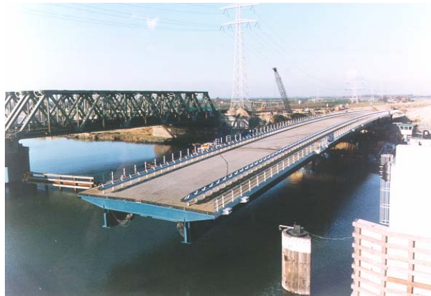
Figure 16 : Bridge in Zuid-Beveland (The Netherlands).
