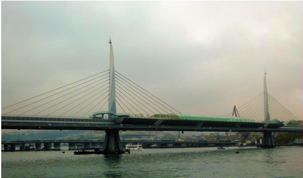
Figure 8. Higher strength weathering steel (A709M HPS485W) in bridge construction. Haliç Metro Bridge in Istanbul, Turkey
