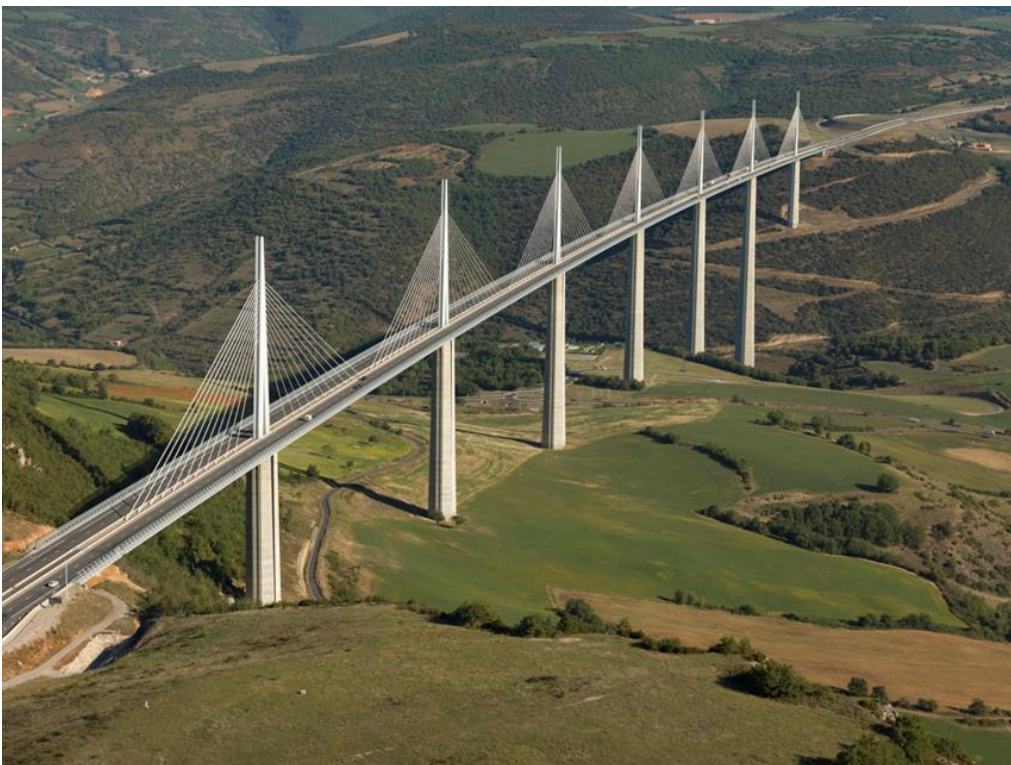
Figure 6. record-breaking: The longest cable-stayed bridge in the world, built with 18.000 t higher strength thermomechanically rolled steel (S460ML).
