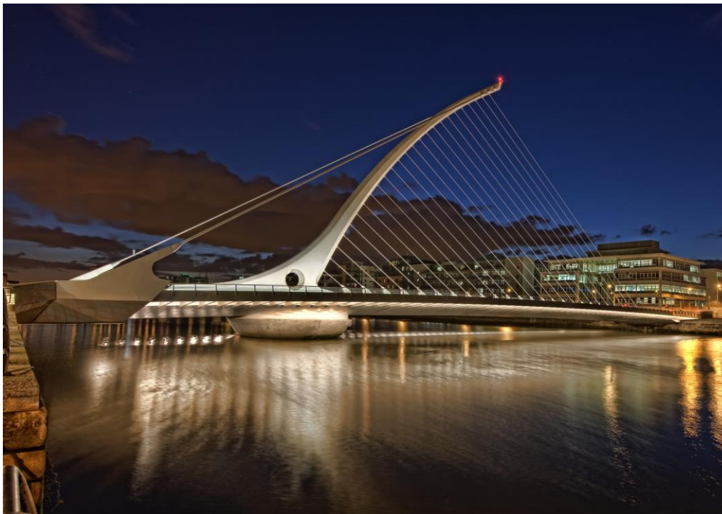
Figure 7. Higher strength quenched and tempered steel (S690QL) in bridge construction. Samuel Becket Bridge in Dublin, Ireland.
