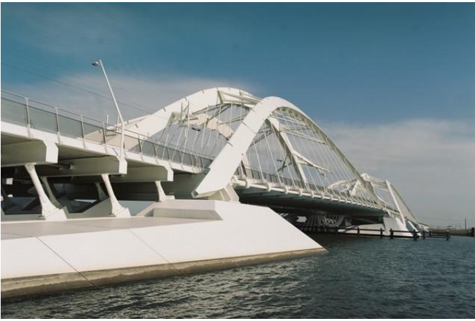
Figure 6. Ennëus-Heerma Bridge in the Netherlands with around 900 t S355M/ML
