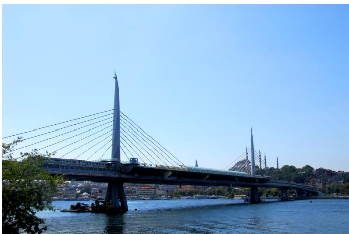
Figure 10. Higher strength weathering steel (A709M HPS485W) in bridge construction. Haliç Metro Bridge in Istanbul, Turkey
