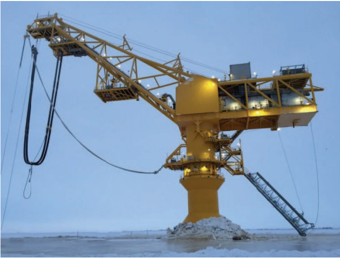
Figure 5. Arctic loading tower in Siberia (Bluewater, 2015). Results of plates with thickness of 65 mm are presented in Figs. 6 and 7.
