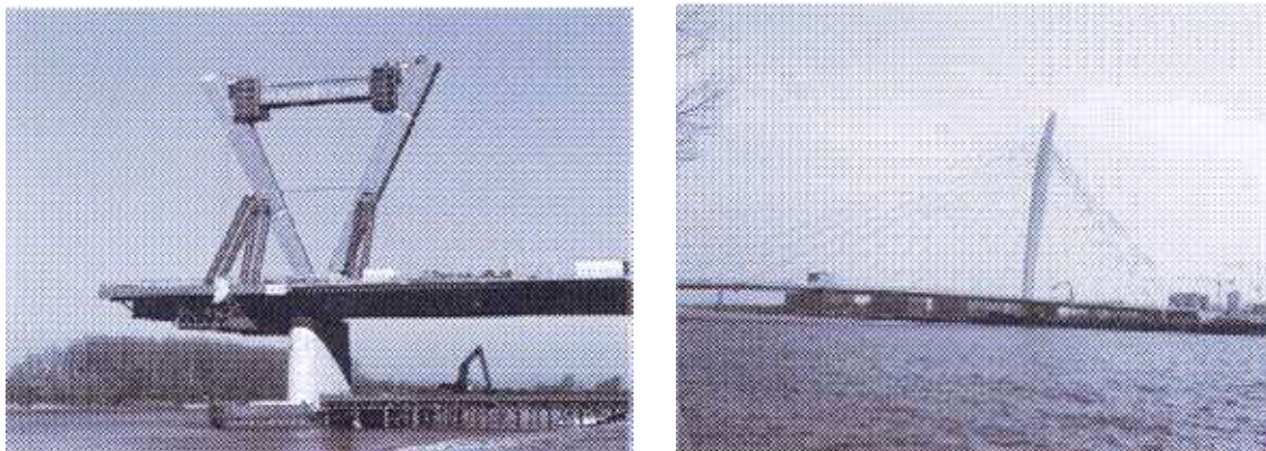
Figure 12: Cable stayed bridges Düsseldorf-North (left) and Prince Claus (right)
