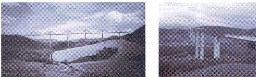
Figure 13: Millau-Viaduct - Future 2005 and current state November 2003
