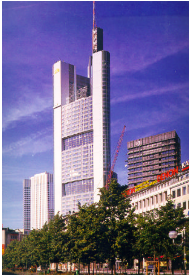
Figure 10: Building construction with heavy plates, Commerzbank-Tower (total view)
