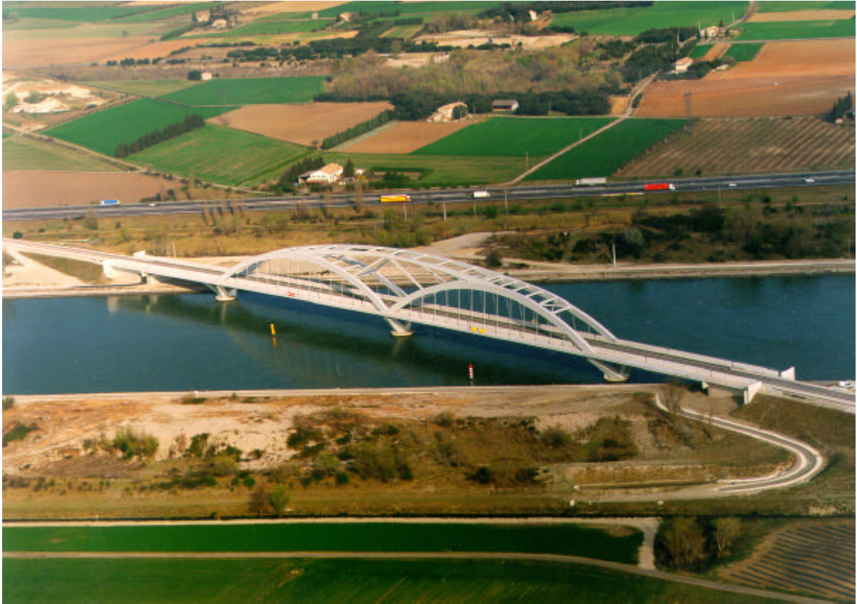
Figure 21: Bridgebuilding with heavy plates, Bridge of Mondragon, F (TGV Méditerranée)
