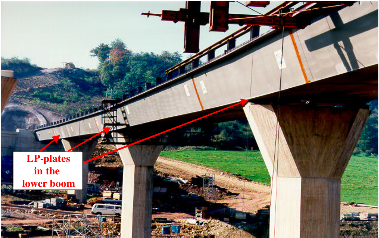
Figure 3: Highway bridge Wellinggen (A8), D
