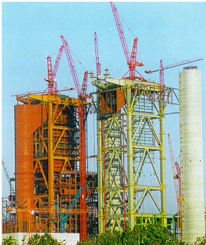
Figure 8: Building construction with heavy plates, power station Schwarze Pumpe
