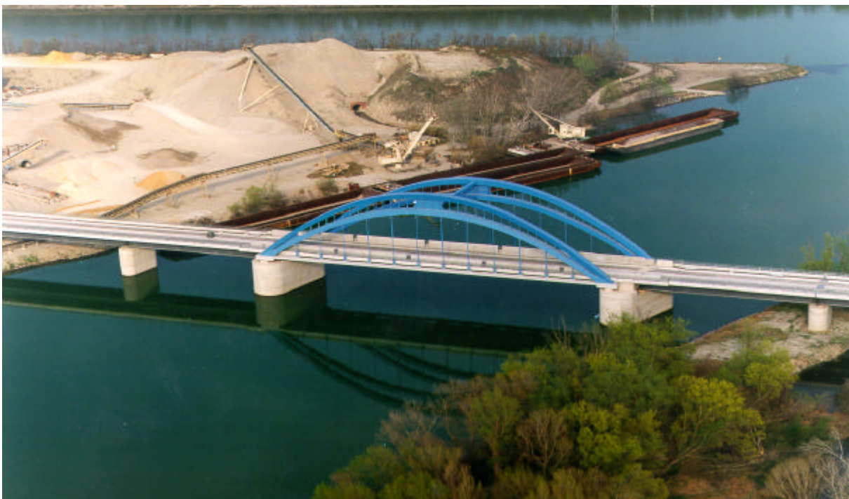
Figure 20: Bridgebuilding with heavy plates, Bridge of Mornas, F (TGV Méditerranée)
