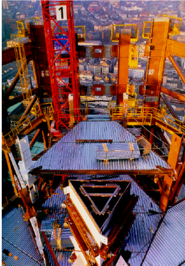
Figure 11: Building construction with heavy plates, Commerzbank-Tower (structure of piles)
