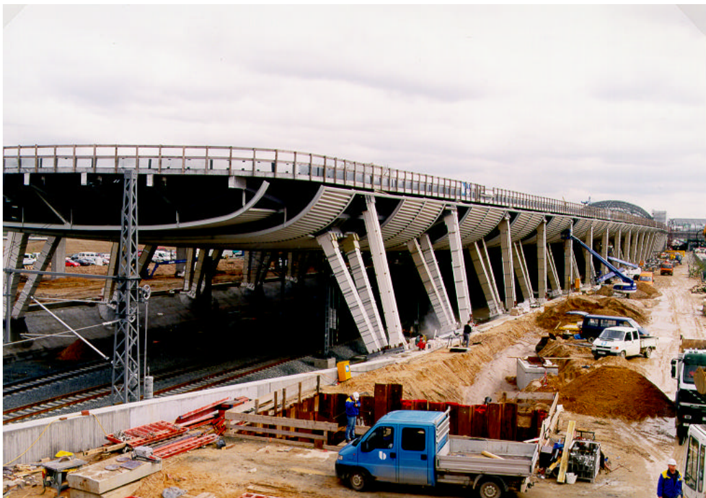
Figure 14: Building construction with heavy plates, High-speed railway station Frankfurt-Airport
