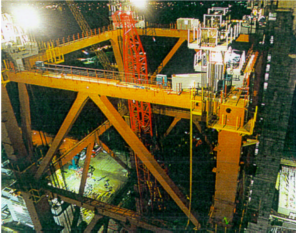
Figure 9: Building construction with heavy plates, power station Schwarze Pumpe
