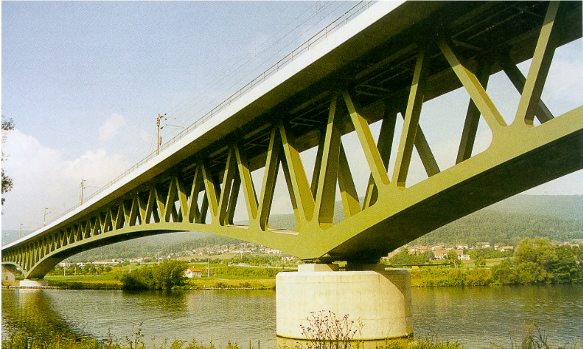
Figure 19: Bridgebuilding with heavy plates, Nantenbachtal-bridge, D
