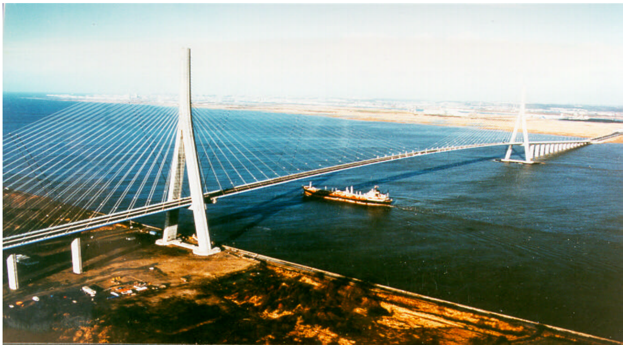
Figure 24: Bridgebuilding with heavy plates, Normandy-bridge, F
