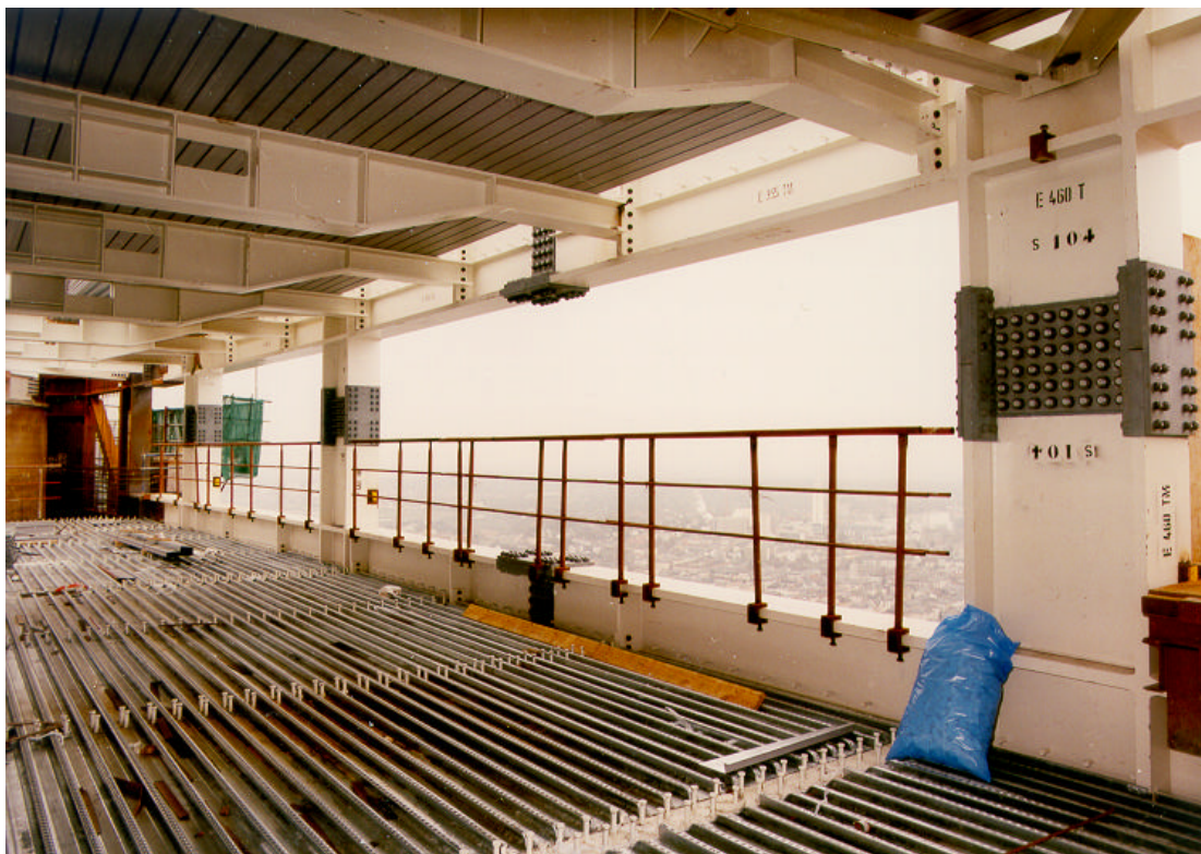
Figure 12: Building construction with heavy plates, Commerzbank-Tower (floor construction)
