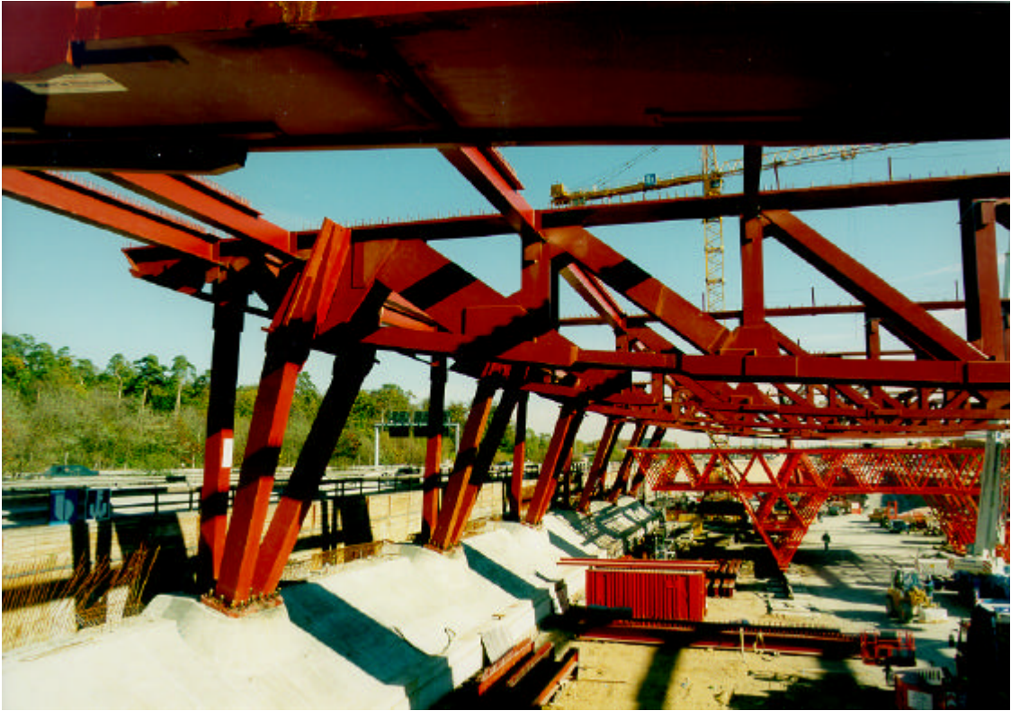
Figure 15: Building construction with heavy plates, High-speed railway station Frankfurt-Airport
