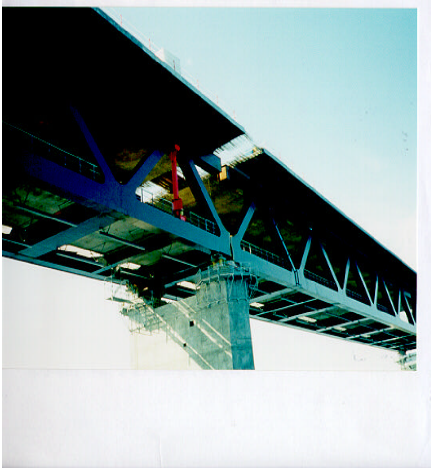
Figure 23: Bridgebuilding with heavy plates, Øresund-bridge, DK-S
