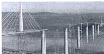
Fig. 5.5.13: Launching with pylon
