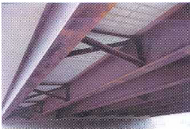
Fig. 18 Weathering steel in the River Tale Bridge (span: 27 m)
