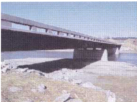
Fig. 20 HPS-70W in bridge next to Springfield, Nebraska
