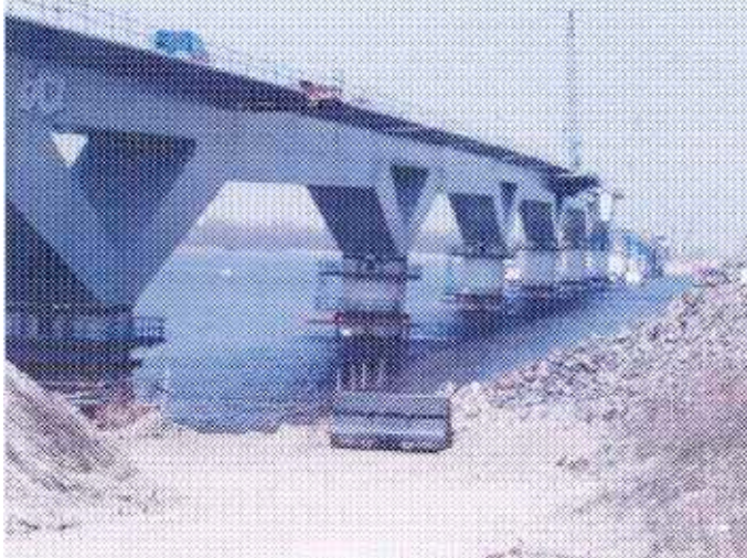
Fig. 2 High-speed railroad bridge Hollandsch Diep
