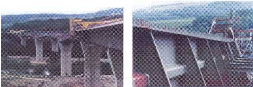
Fig. 8 LP-plates in the upper flange of the Schengen bridge
